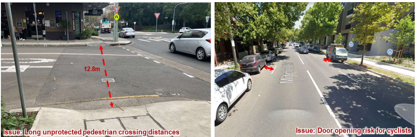
Figure 3.1: Safety Issues Due to the Road Environment (Mitchell Road, Harley to Maddox)
