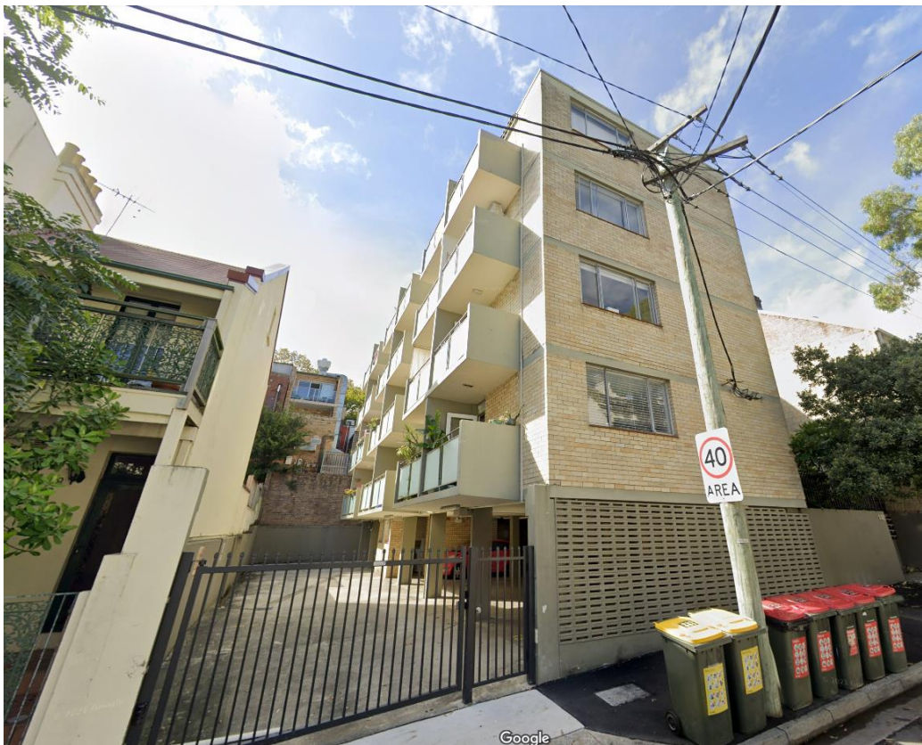
Figure 3. 100-104 Brougham Street looking east from Brougham Street
